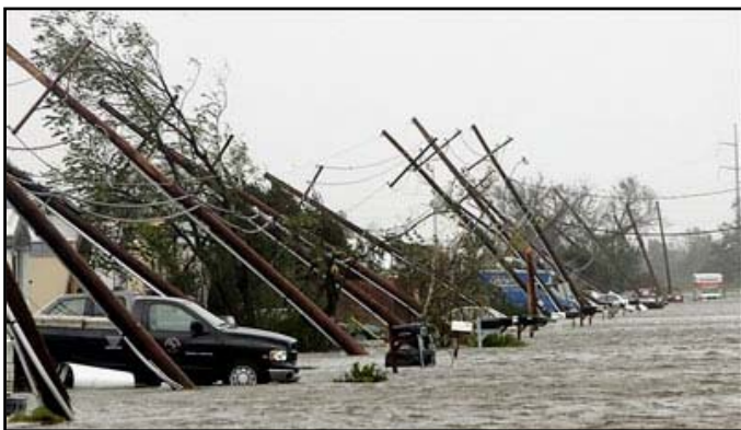
Power lines damaged by hurricane Katrina
