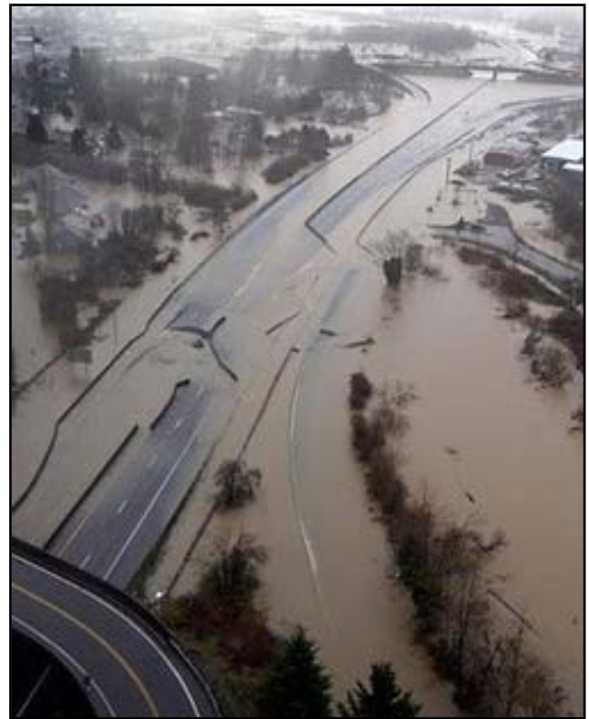
Aerial view of flooding on Interstate 5 [Photos courtesy Jeremy King]
