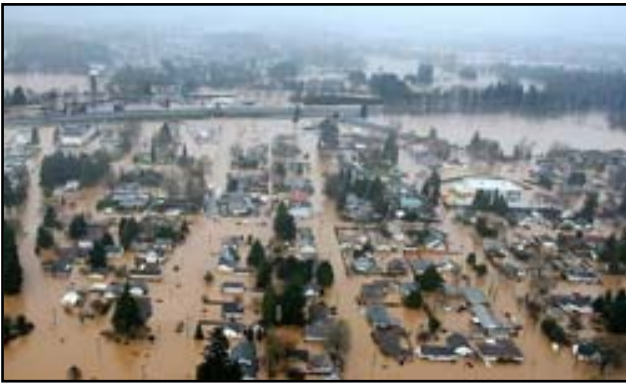
The town of Chehalis, Washington, almost totally submerged by water
